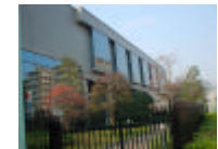
SECOM Data Center in 2001
